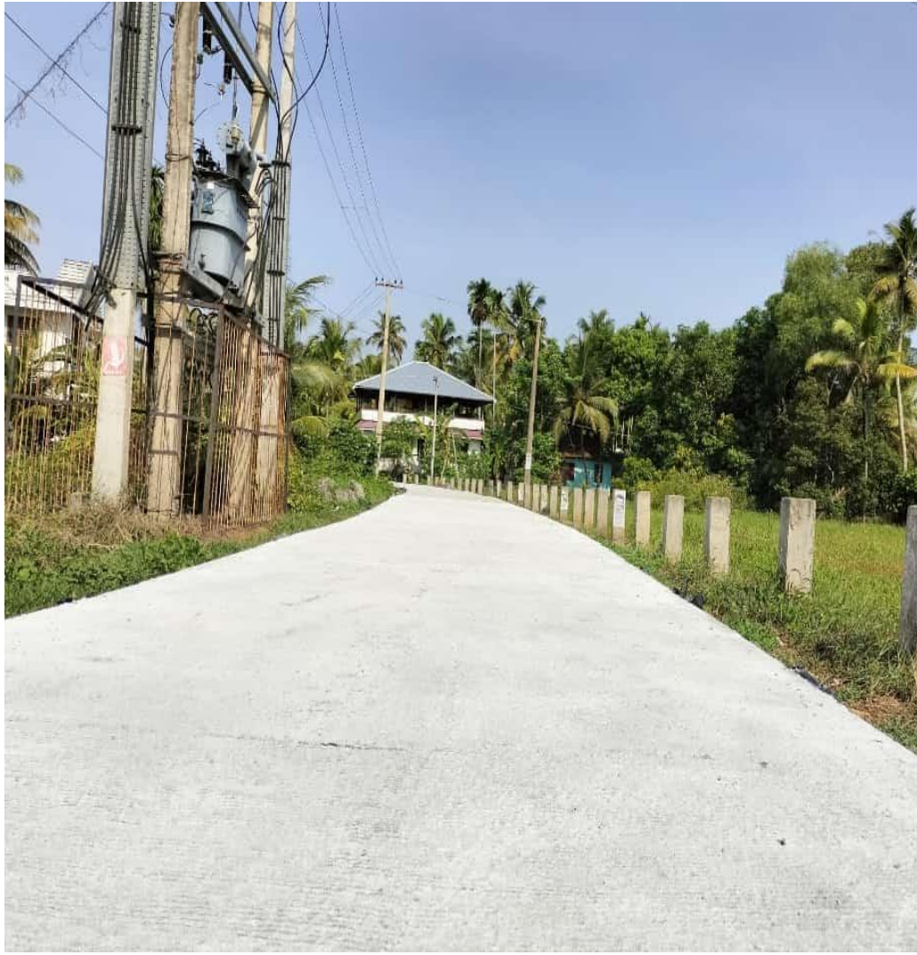
Kavumpadi to Perumal Jetty Road, Alappuzha
