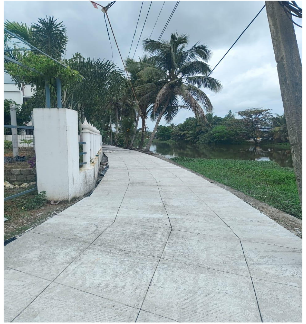
Pekkali Bridge to Kadakom Road, Alappuzha
